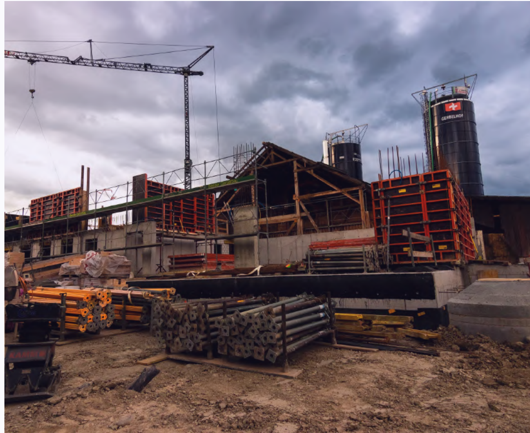
CONSTRUCTION MATERIALS FACULTY OF ENGINEERING
